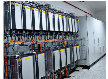
Automation was sub-contracted to Dutch specialist Beenen (photo: IDM)
