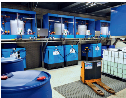
Together with Diversey, ALPMA also supplied the CIP lines for the new RO plant (photo: IDM)
